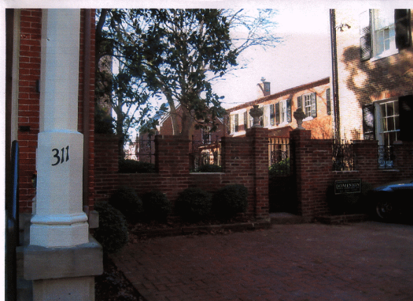
Figure 1: View from S St. Asaph Street
