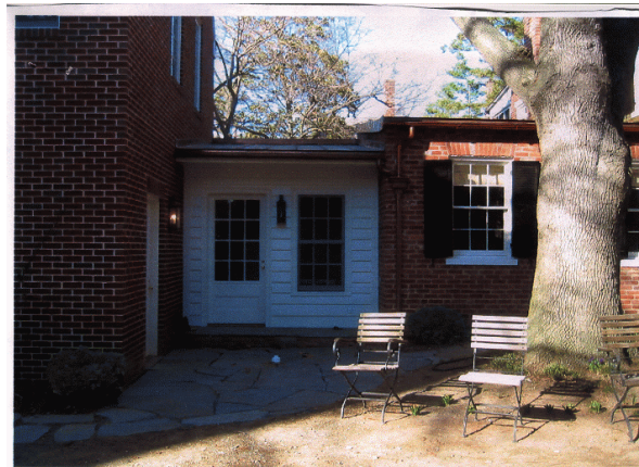
Figure 2: View of Addition from Side
