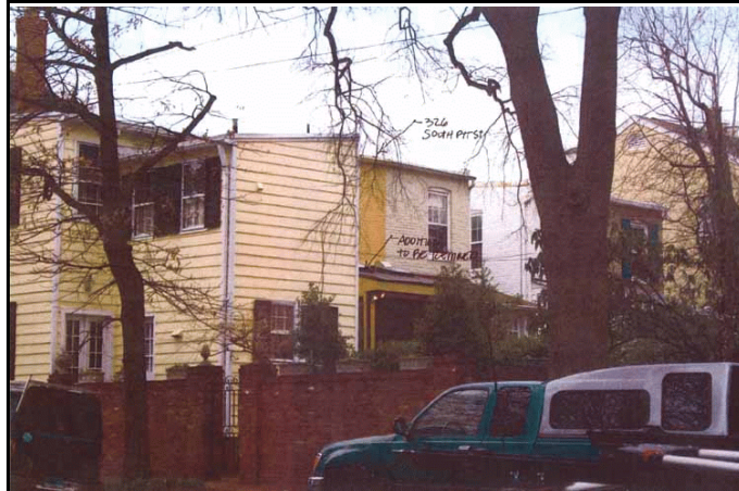
Figure 2 View from Wolfe Street
