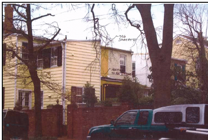
Figure 2 View from Wolfe Street
