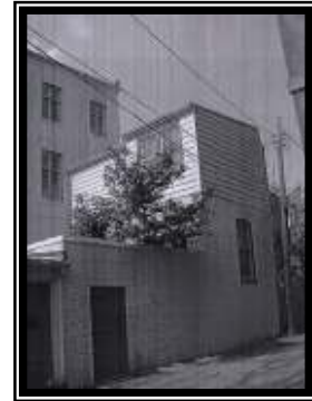
Figure 3 Rear Portion to be demolished
