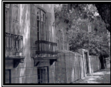
Figure 2 Garden wall facing Prince Street
