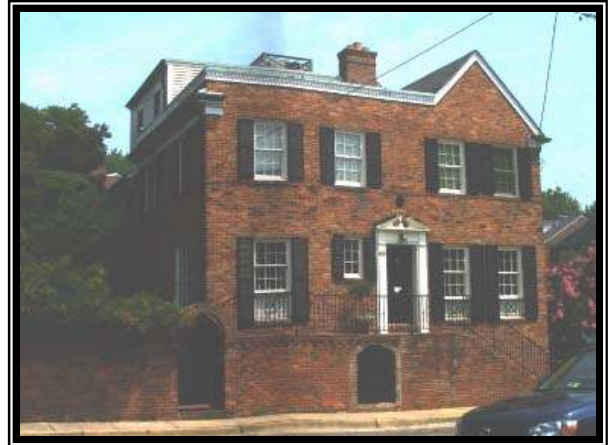
Figure 2 - View of west and south elevations
