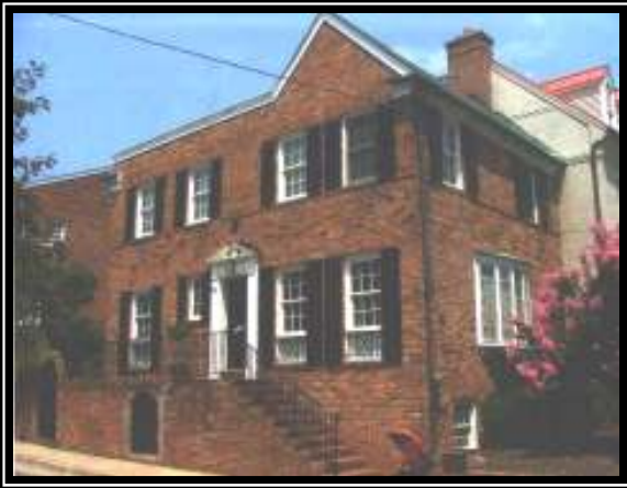
Figure 1 - View of south and east elevations
