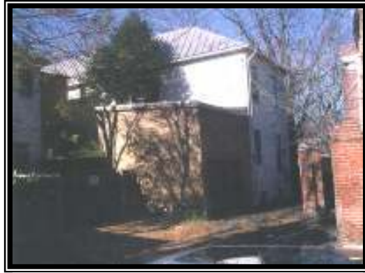
Figure 2 - View of garage
