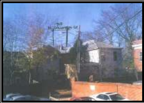
Figure 1 - View of east (rear) elevation
