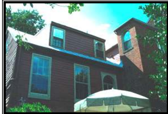
Figure 2 - Upper portion of east elevation
