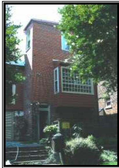
Figure 5 - Northern end of east elevation
