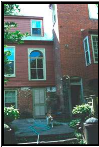
Figure 4 - Center section of east elevation
