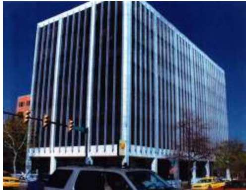
Figure 1 -1 Existing Jefferson Building at 901 North Washington St
