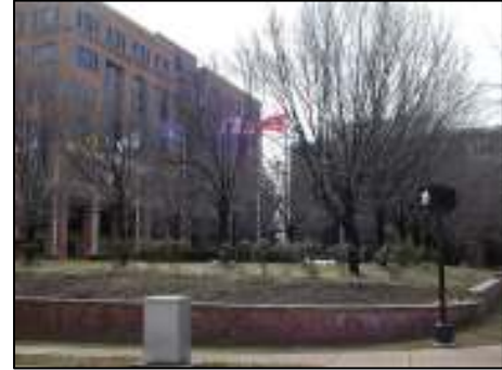
Figure 8: Existing AFBA Building
