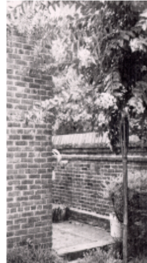
Figure 3 - Rear at side yard
