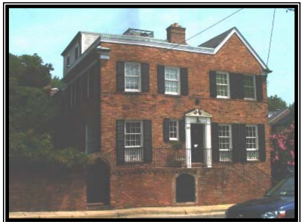
Figure 2 - View of west and south elevations
