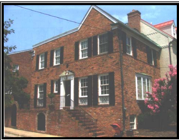
Figure 1 - View of south and east elevations
