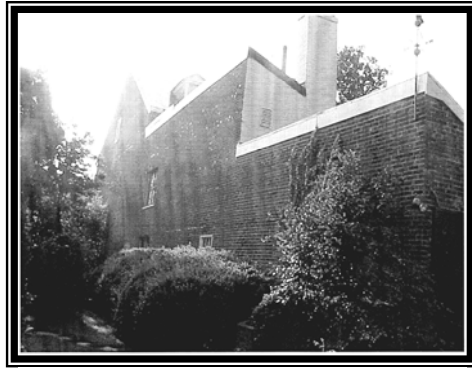
Figure 2 - North elevation of rear ell
