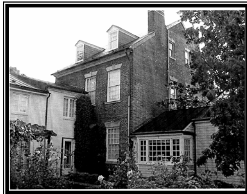
Figure 3 - North elevation of main block
