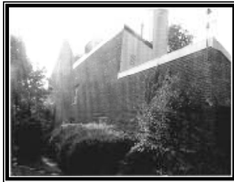
Figure 2 - North elevation of rear ell
