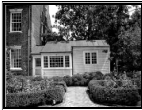
Figure 1 - West elevation of kitchen wing
