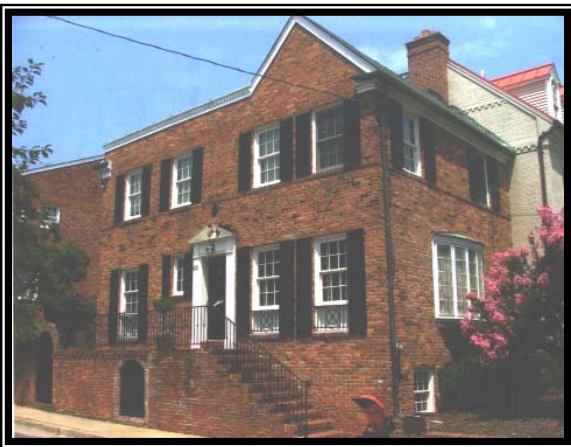
Figure 1 - View of south and east elevations
