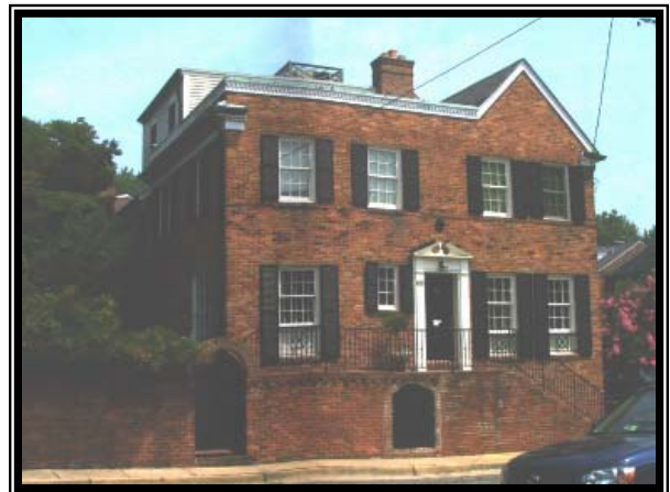
Figure 2 - View of west and south elevations
