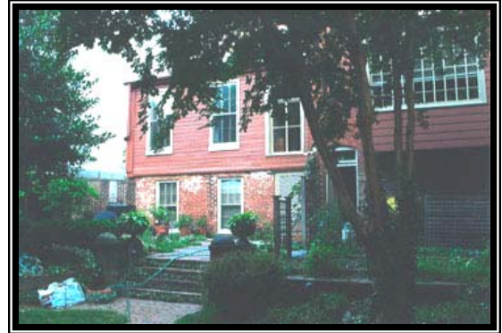
Figure 2 - Upper portion of east elevation
