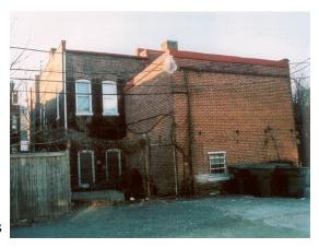
rear of the building will be removed and the openings infilled with brick to match. A series of four white finished canister lights will be installed at the top of the first story along the south elevation. Views of this section of the building are limited.
