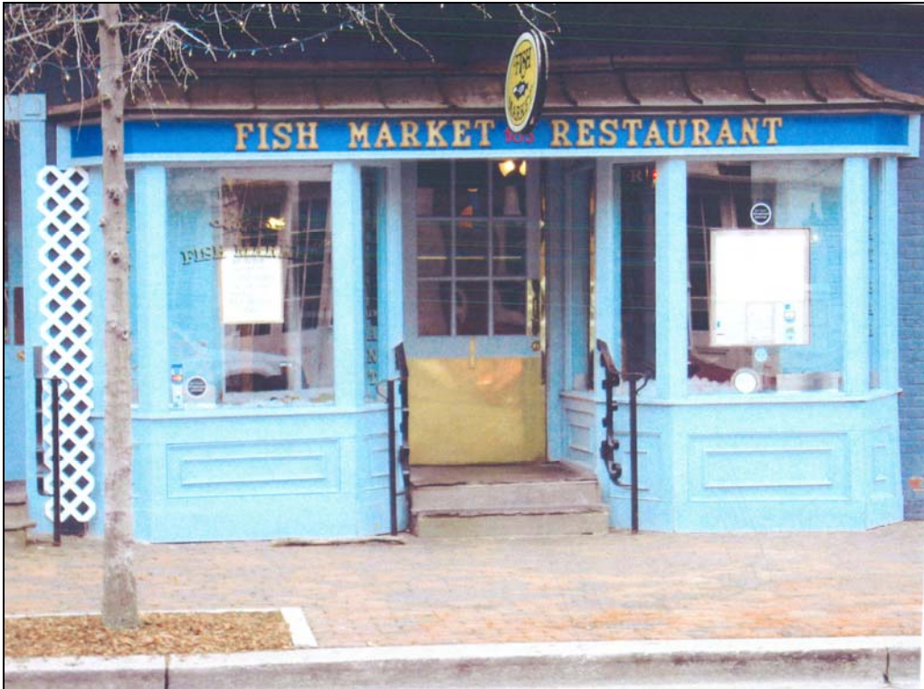
Figure 1. Existing storefront, 105 King Street.
