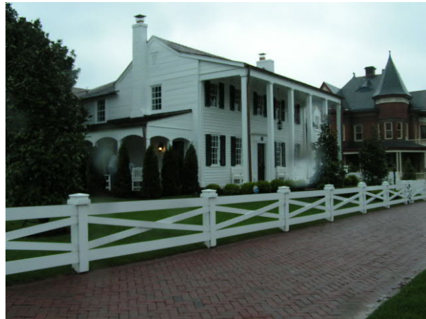
Figure 7 New Perimeter Fencing
