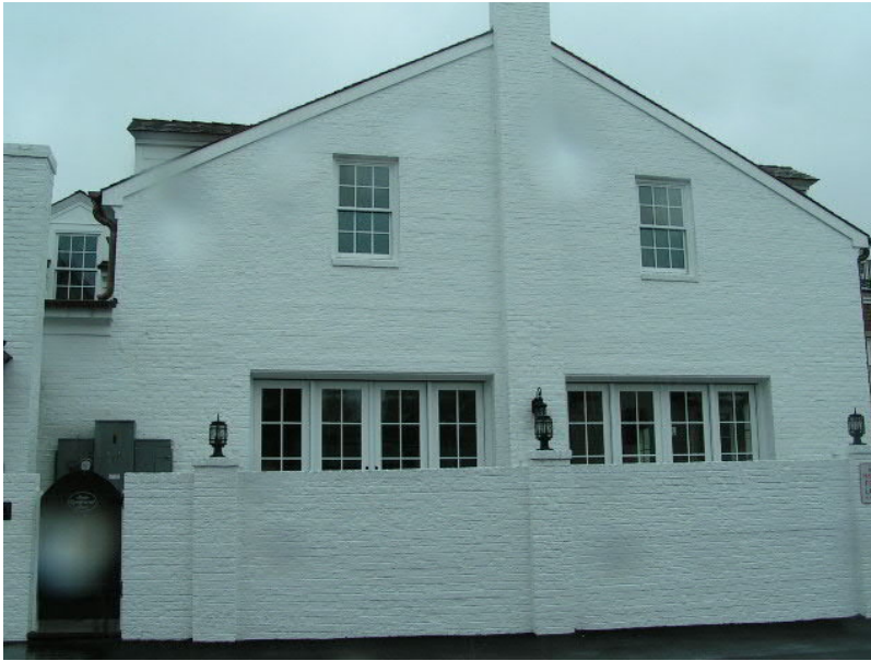
Figure 8 New Pier and Wall Lights
