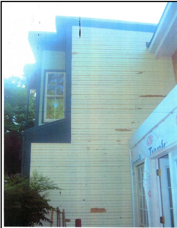
Figure 2 East Wall of Addition
