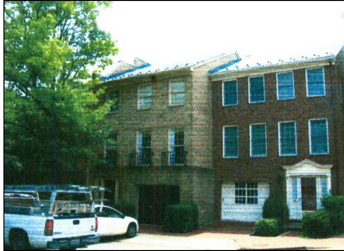
Figure 1. Front elevation of 124 Quay (left).
