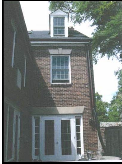
Figure 2: Area of demolition/encapsulation
