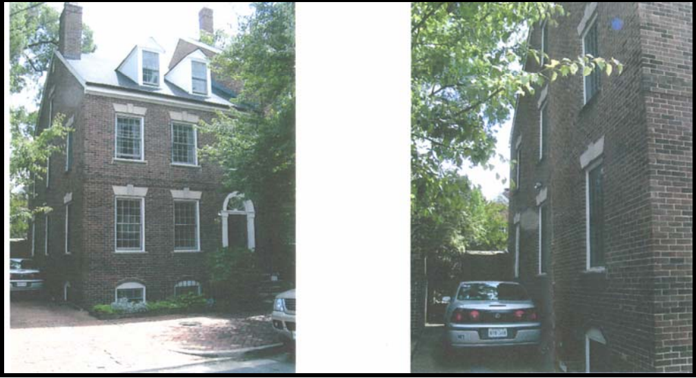
Figure 2: Photo of existing front and side elevations
