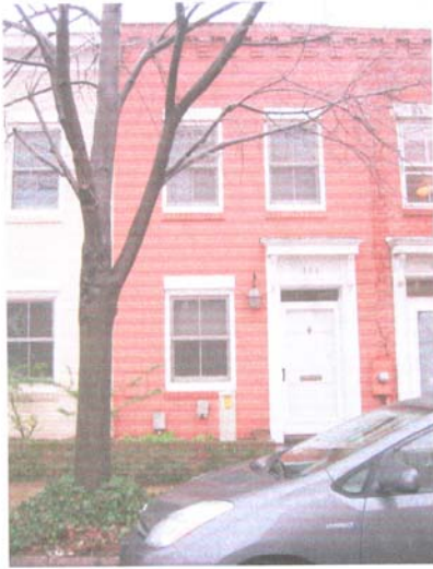
Front View of 334 Commerce St.
