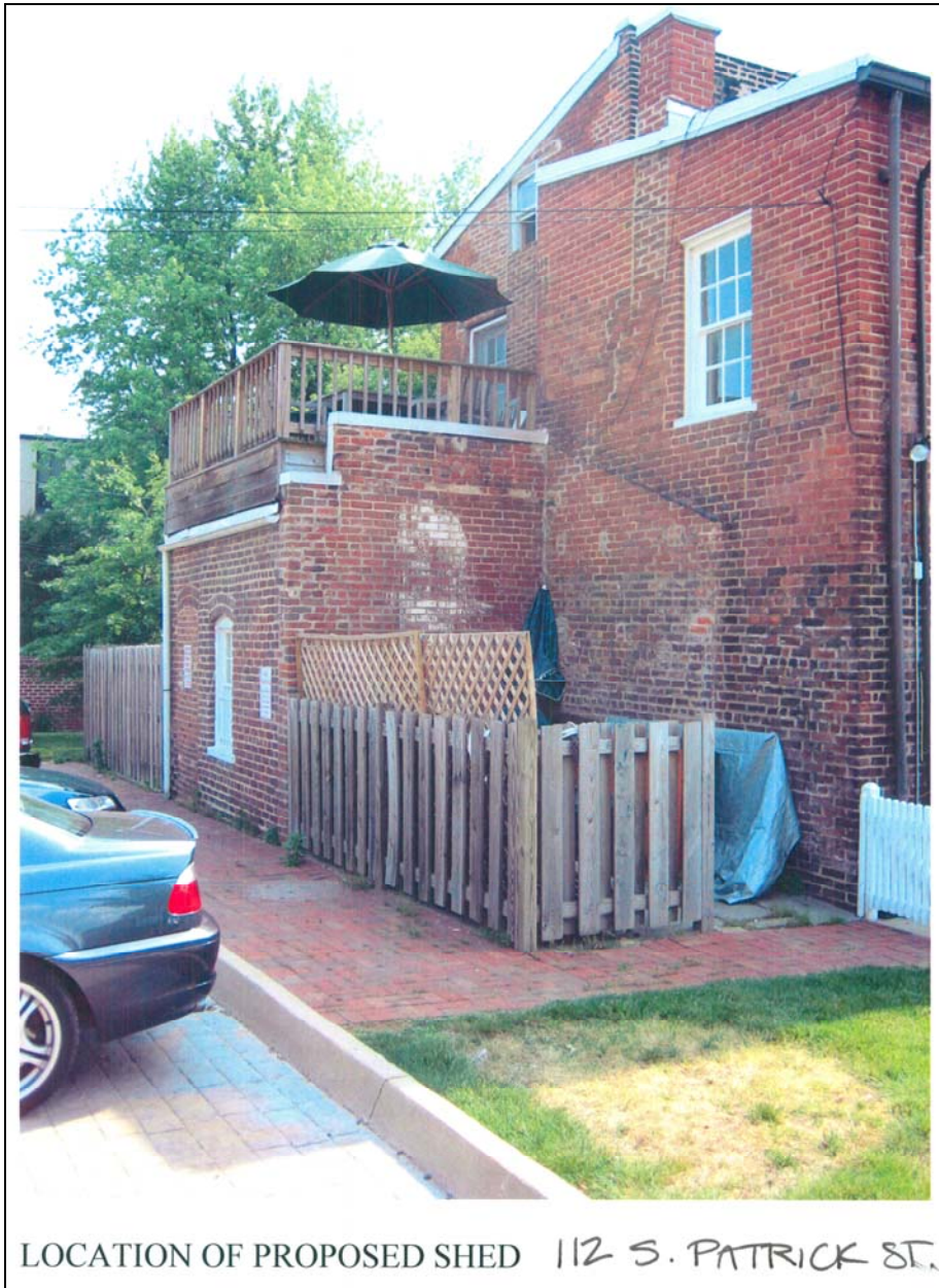
Figure 2: Existing photo of proposed shed location.
