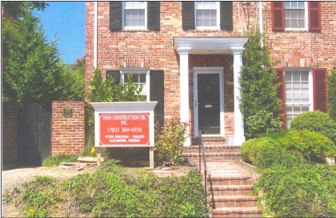
Figure 2. 809 South Royal Street front yard and façade.
