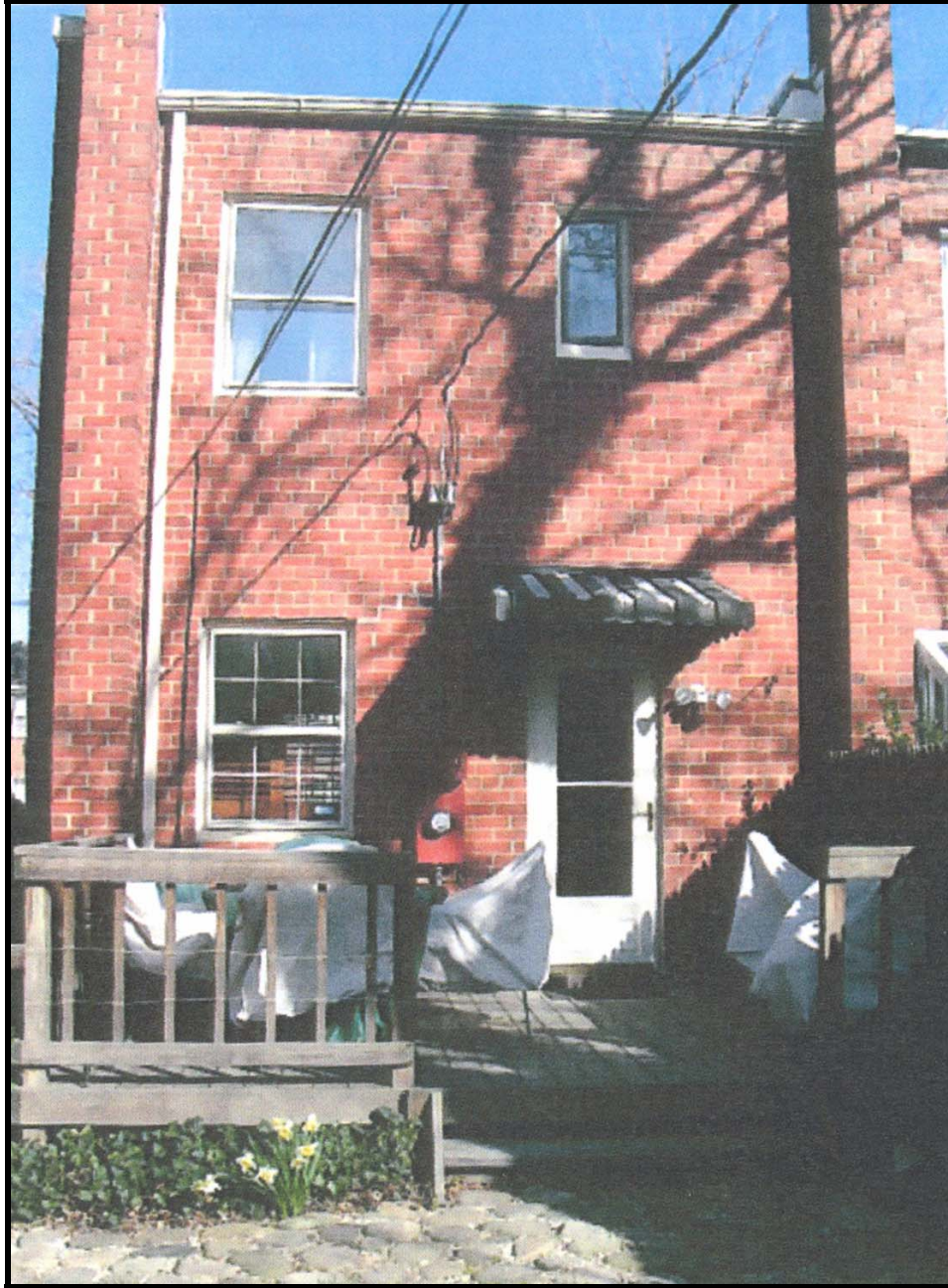
Figure 2: Photo of rear elevation
