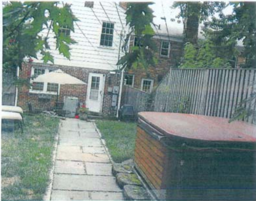
Two story addition at 900 block of S. Columbus (only addition in row)
