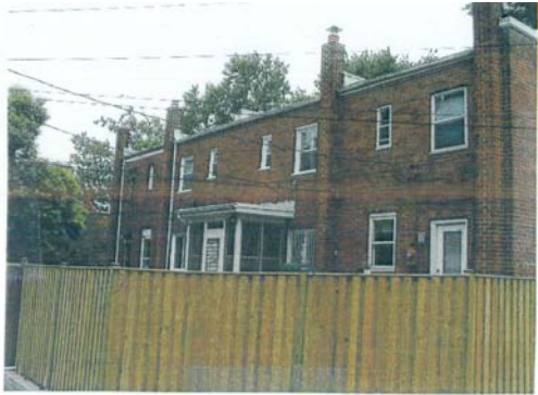
Addition at house at 800 block of Jefferson Street (alley behind 725 S. Columbus Street)
