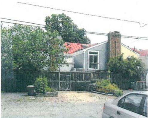
Two story addition at row houses of 800 block of S. Columbus Street
