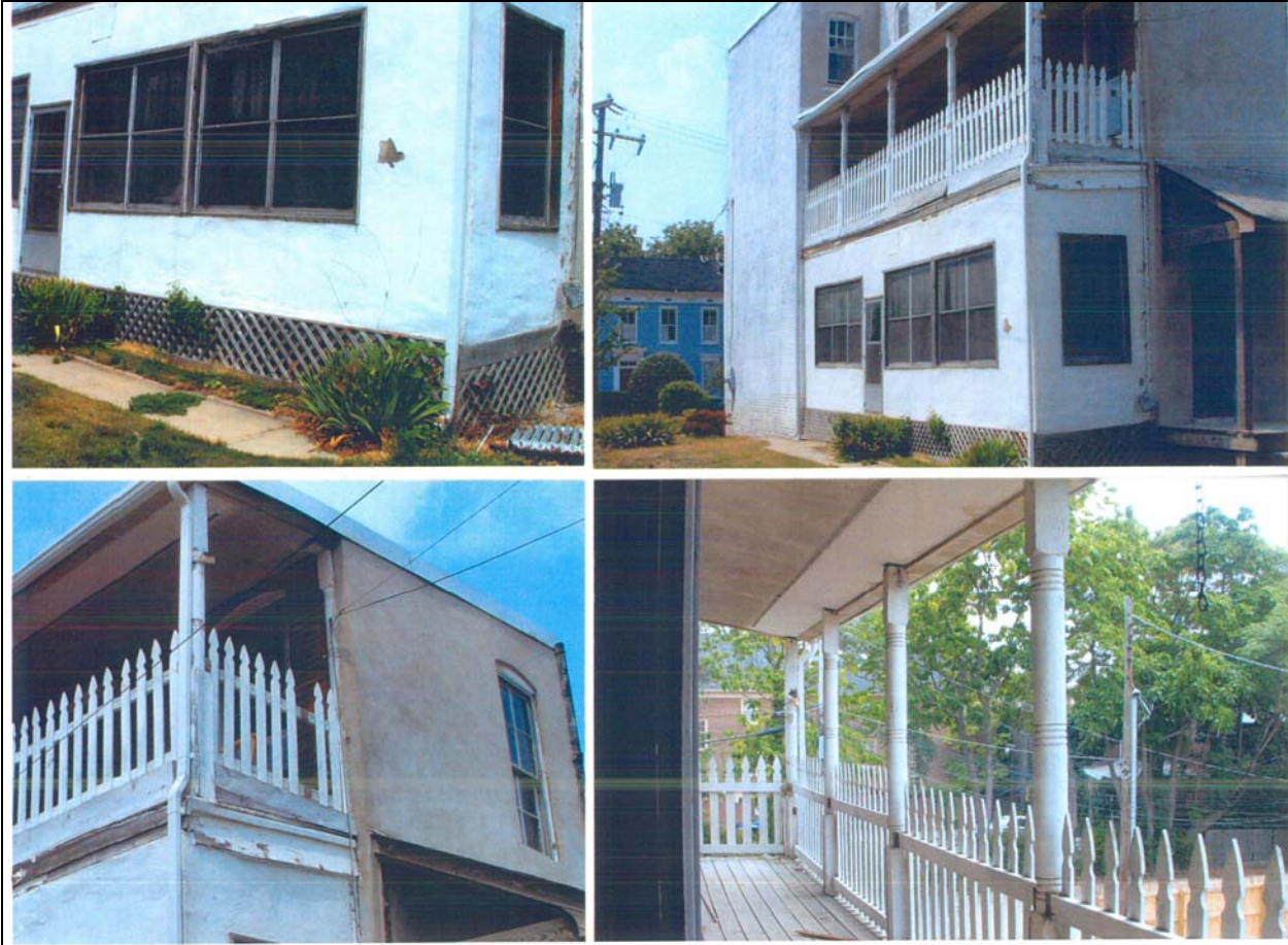
Figure 3. Existing two-story porch on south elevation, to be replaced.
