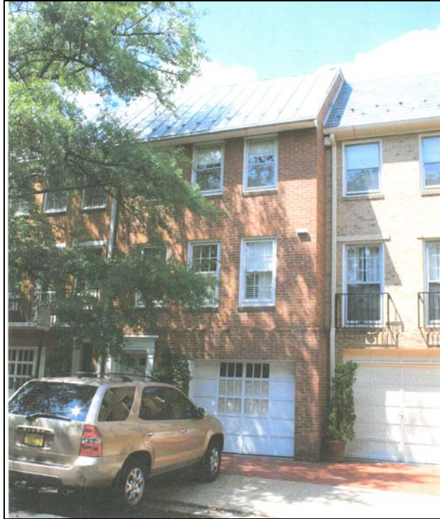
Figure 2. Front (south) elevation.
