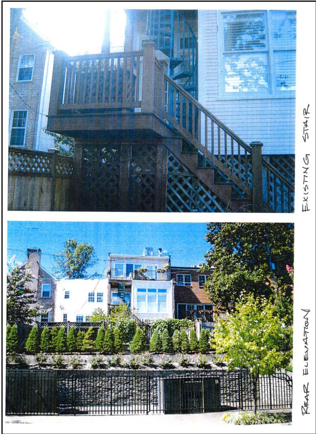
Figure 1 Existing Rear Elevation
