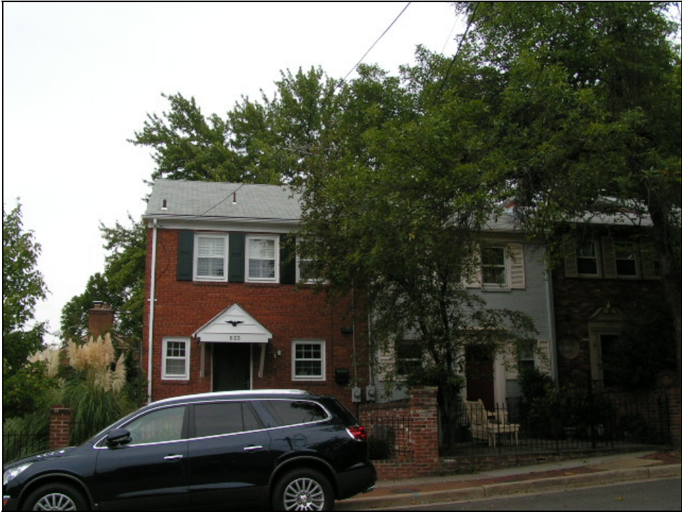
Figure 1. Front (east) elevation of 833 South Fairfax Street.
