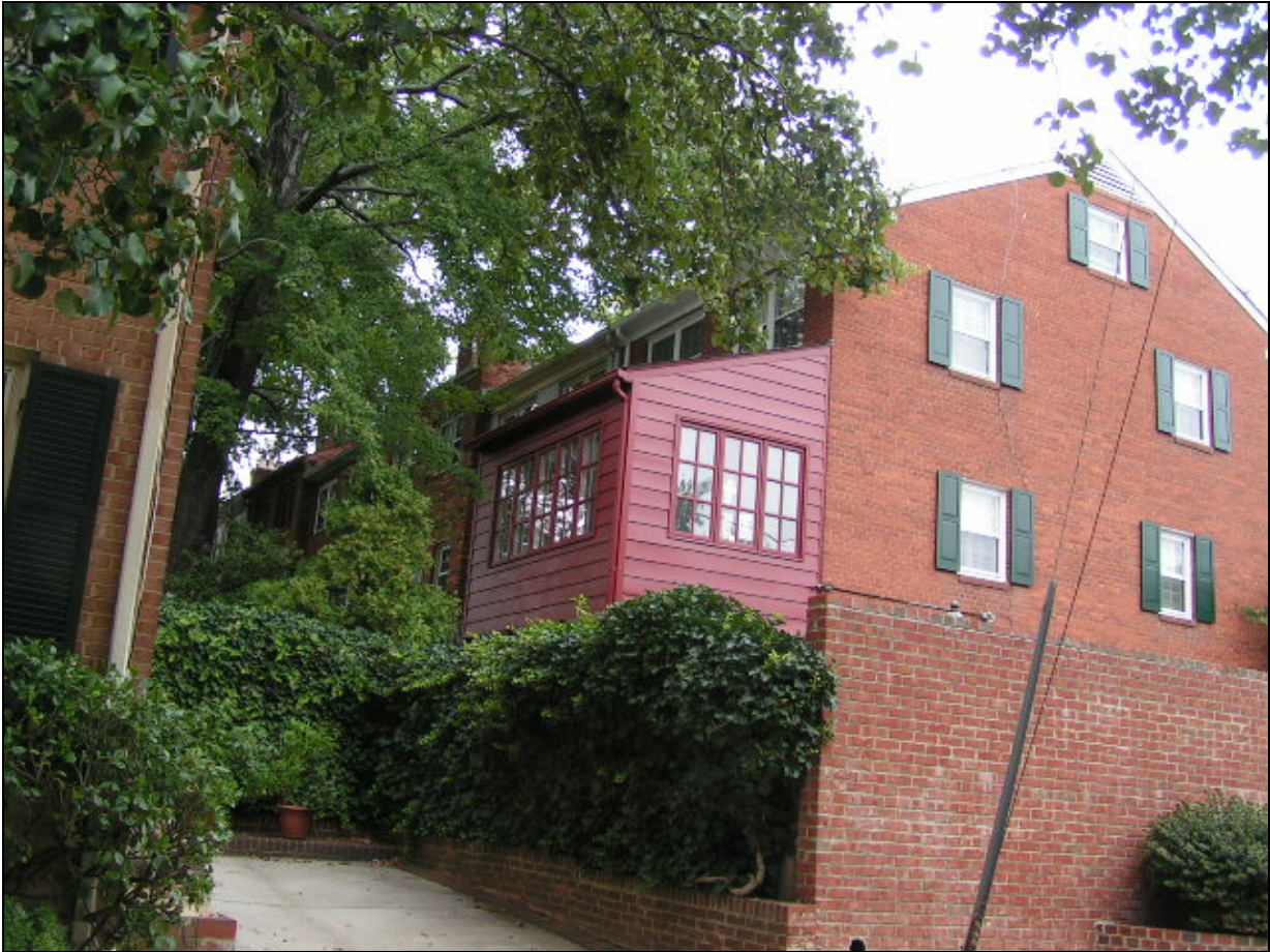
Figure 3. Rear (west) and side (south) elevations.
