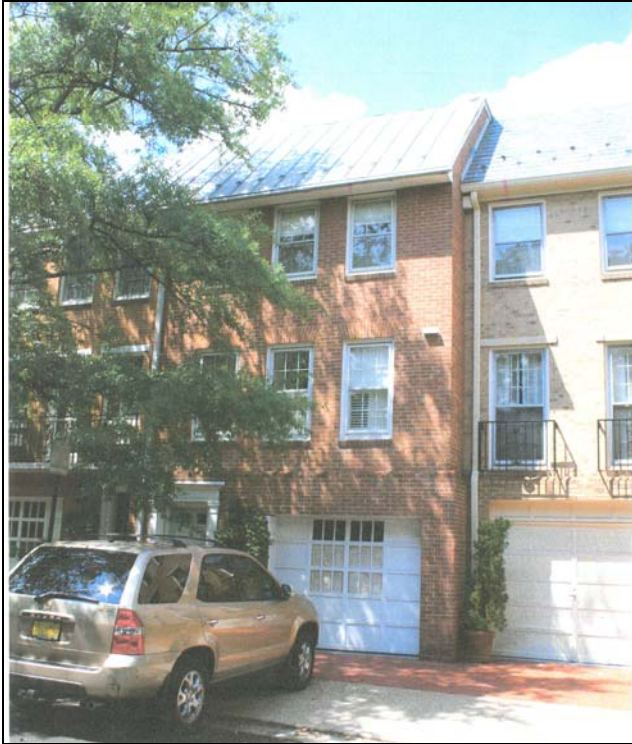
Figure 2. Front (south) elevation.
