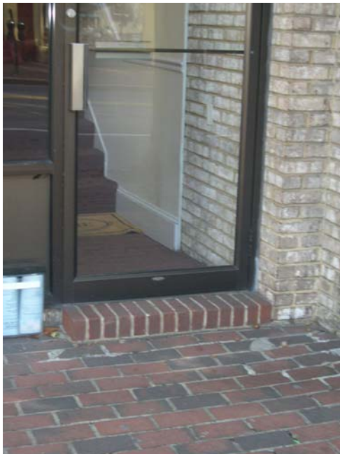
Detail of Brick Stoop to be Removed
