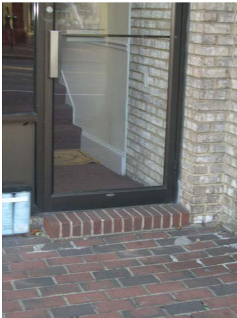
Detail of Brick Stoop to be Removed
