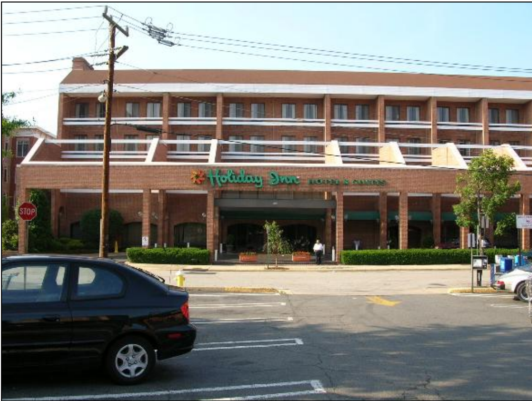
Figure 3. Existing conditions at 625 First Street, south elevation.
