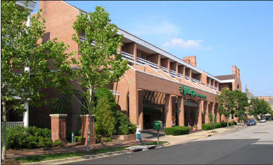
Figure 2. Existing conditions at 625 First Street.
