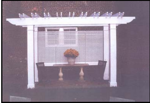
Figure 8: Front View of Arbor as Built
