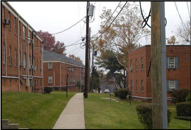
Figure 4: Existing Hunting Terrace Site
