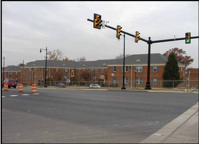
Figure 3: Existing Hunting Terrace Site
