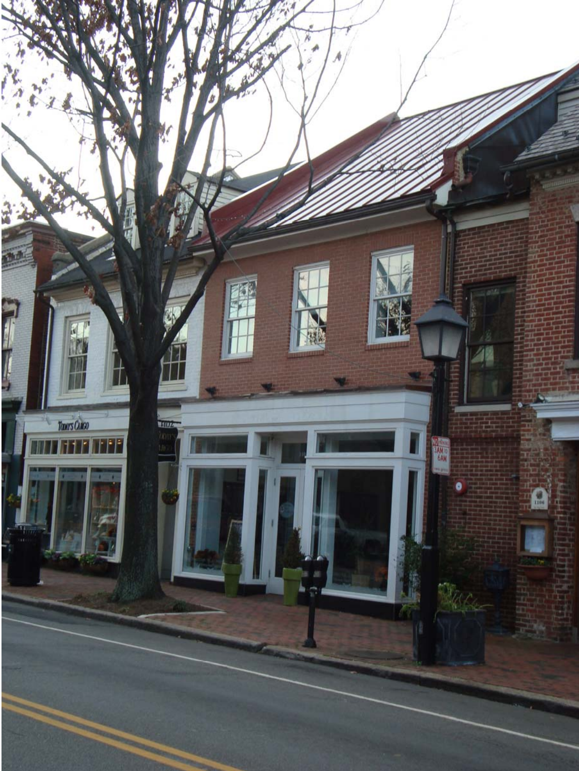
Existing Storefront showing adjacent properties
