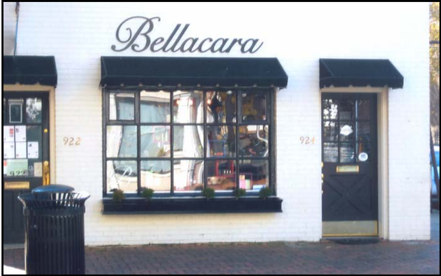
Figure 1 Existing King Street Facade
