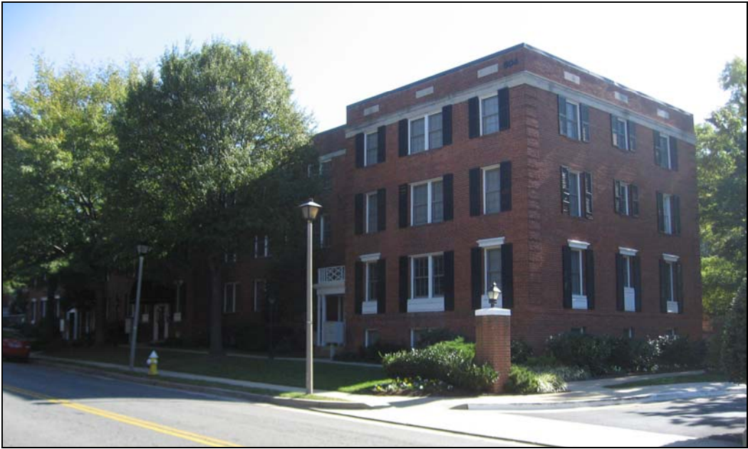
Figure 1. Existing conditions, Bashford Lane.
