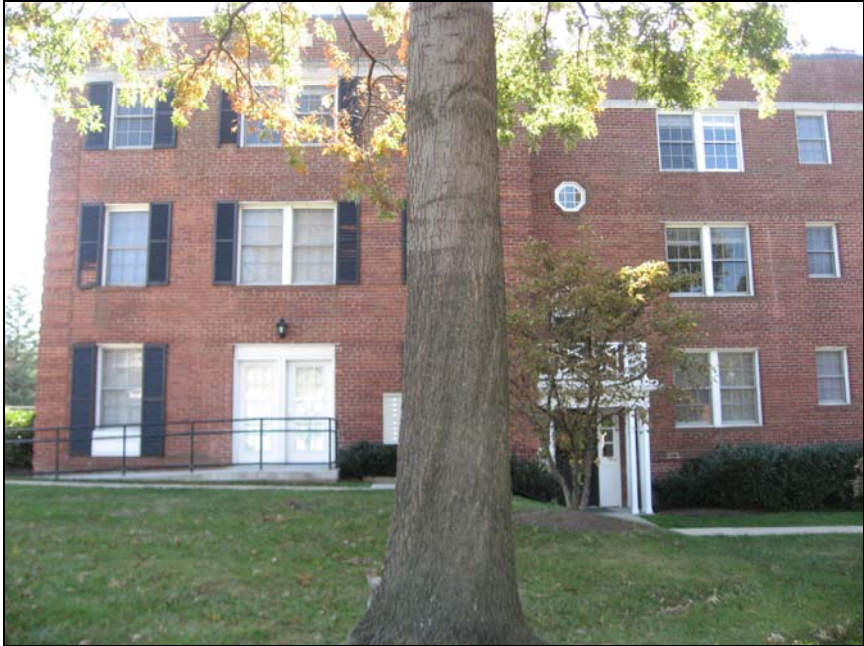
Figure 3. Existing conditions on Bashford Lane, showing windows with and without shutters.
