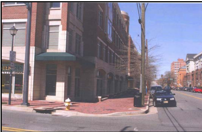
Figure 4: Door at the Corner of Pendleton Street and St. Asaph Street
