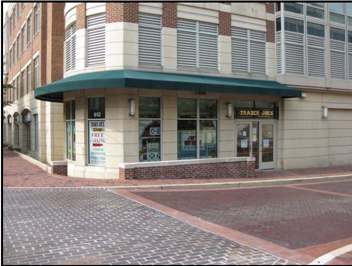
Figure 1: Existing Window and Entrance Only Door at St. Asaph Street
