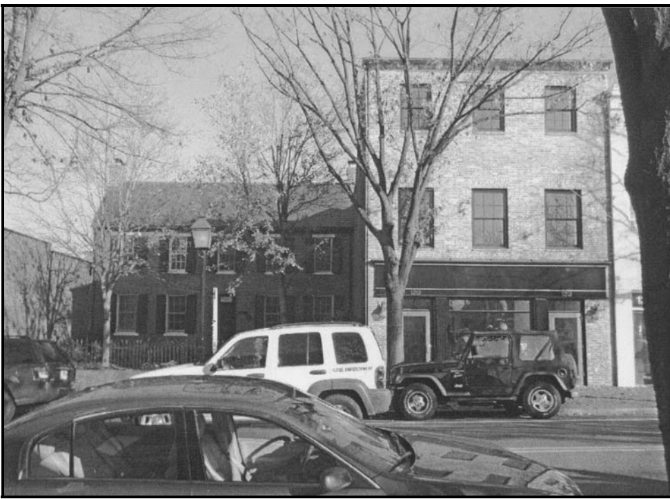
Figure 4: Buildings Located Across King Street
