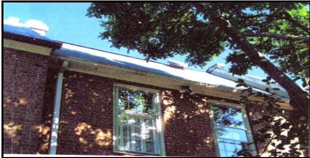
Figure 3: Existing Rear Elevation
