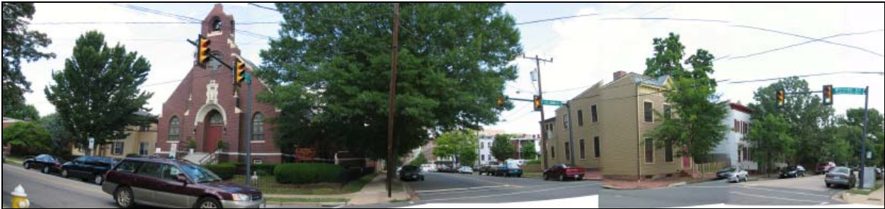
Figure 2. Looking southeast toward site from North Columbus Street, with St. Joseph's Church on left.
