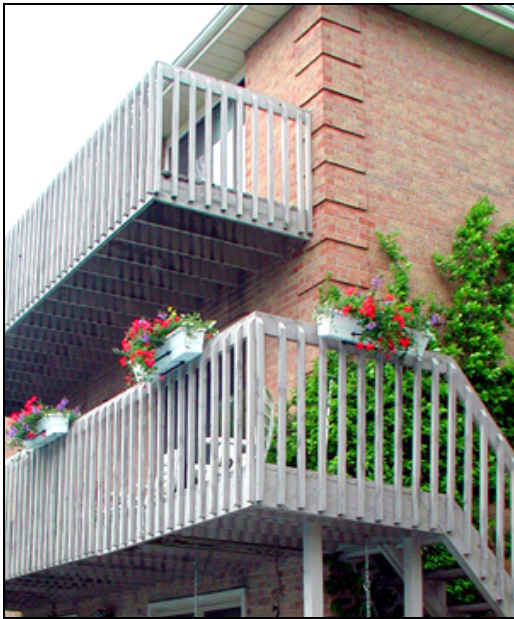
Figure 7: "Notched" Picket Balustrade
