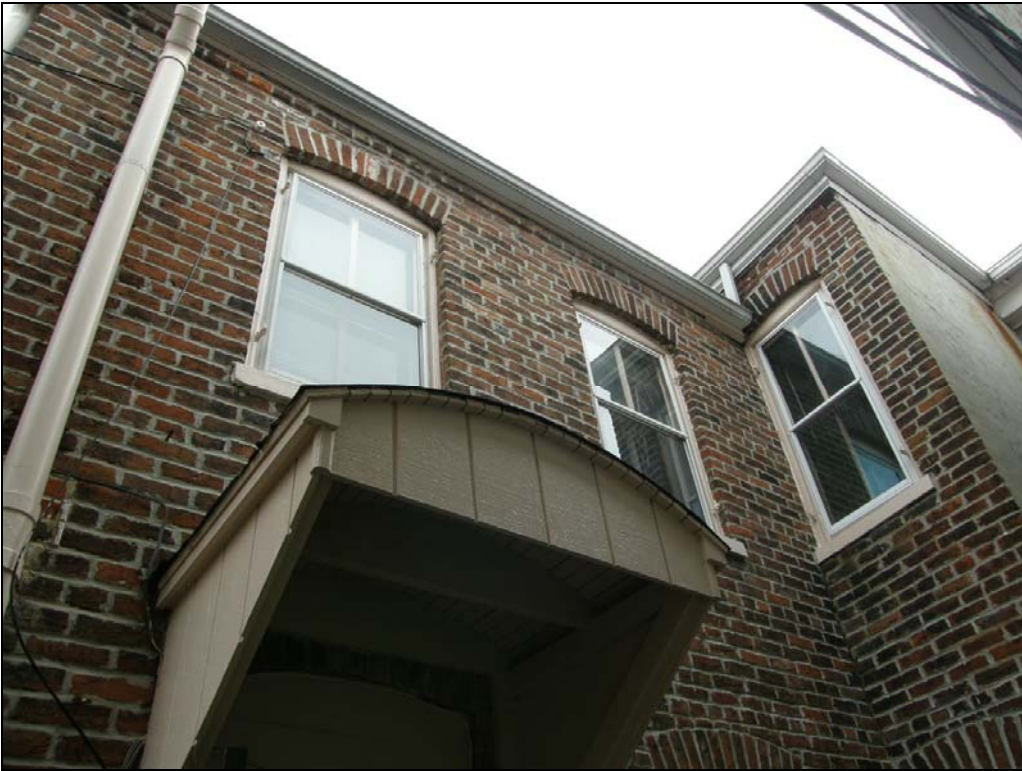
Figure 5: Detail Rear (West) Elevation
