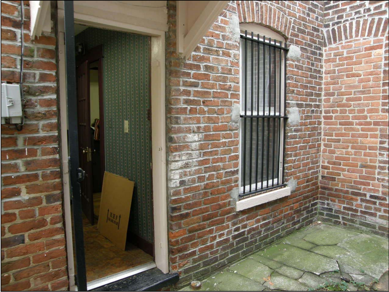
Figure 6: Detail Rear (West) Elevation
