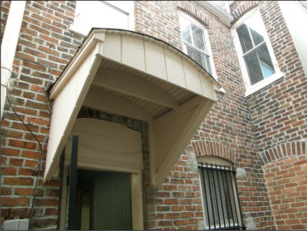
Figure 4: Detail Rear (West) Elevation
