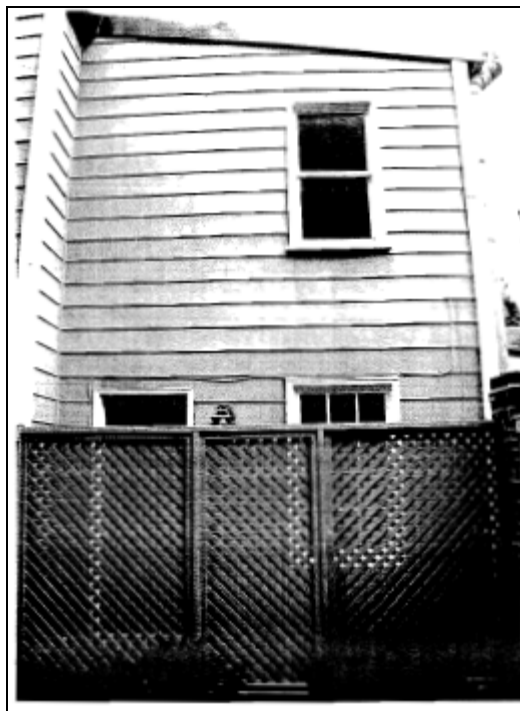
Figure 3. South elevation of rear ell.
