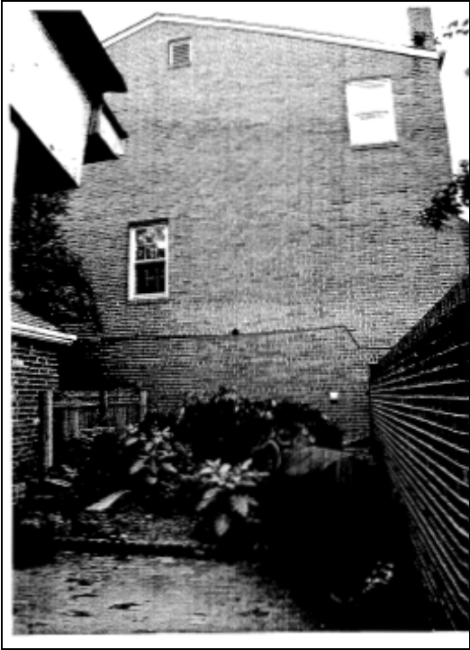
Figure 5. Rear yard, looking eastward.
