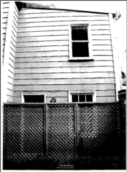
Figure 3. South elevation of rear ell.
