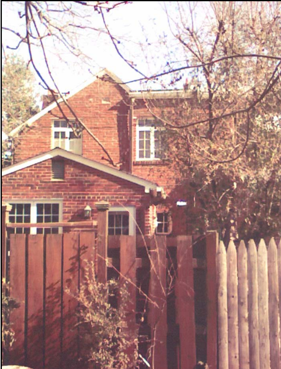
Figure 1: Photograph of Existing Rear Façade
