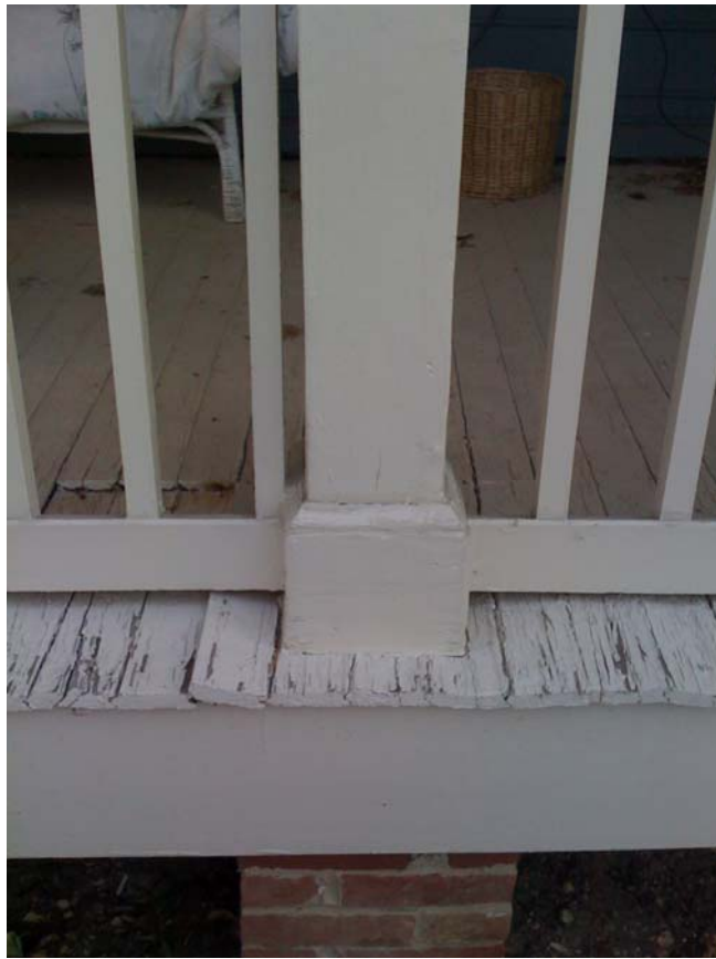
Figure 8: Detail View of Porch Post
