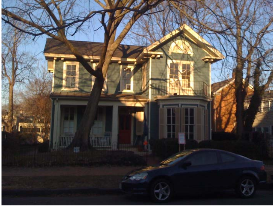
Figure 1: Front Elevation of Dwelling
