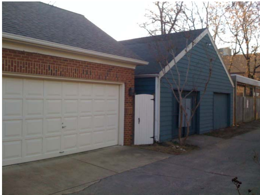
Figure 4: Alley View of Outbuilding with View of Adjacent Neighbor's Garage
